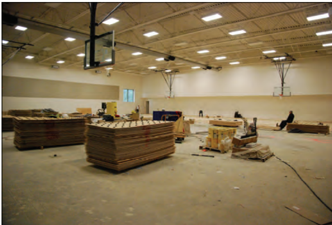
Upper auxiliary gym wood floor installation underway.
