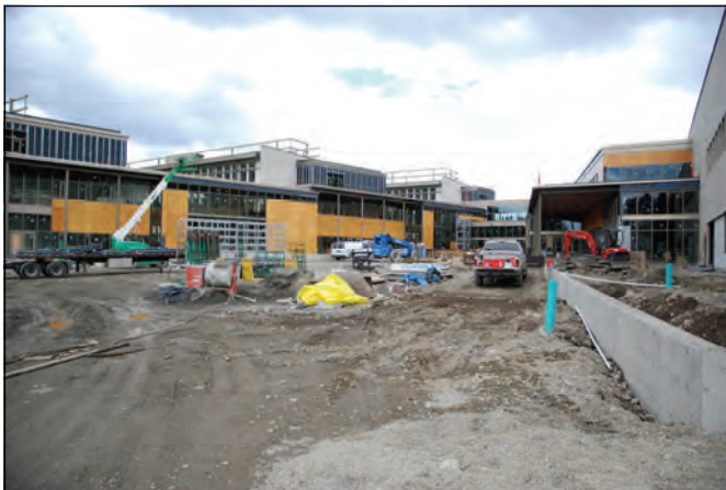
Central Plaza—seat wall formed and poured.
