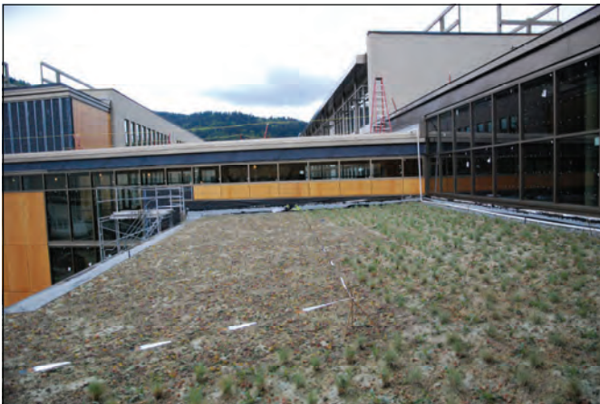
Green roof outside the Library.
